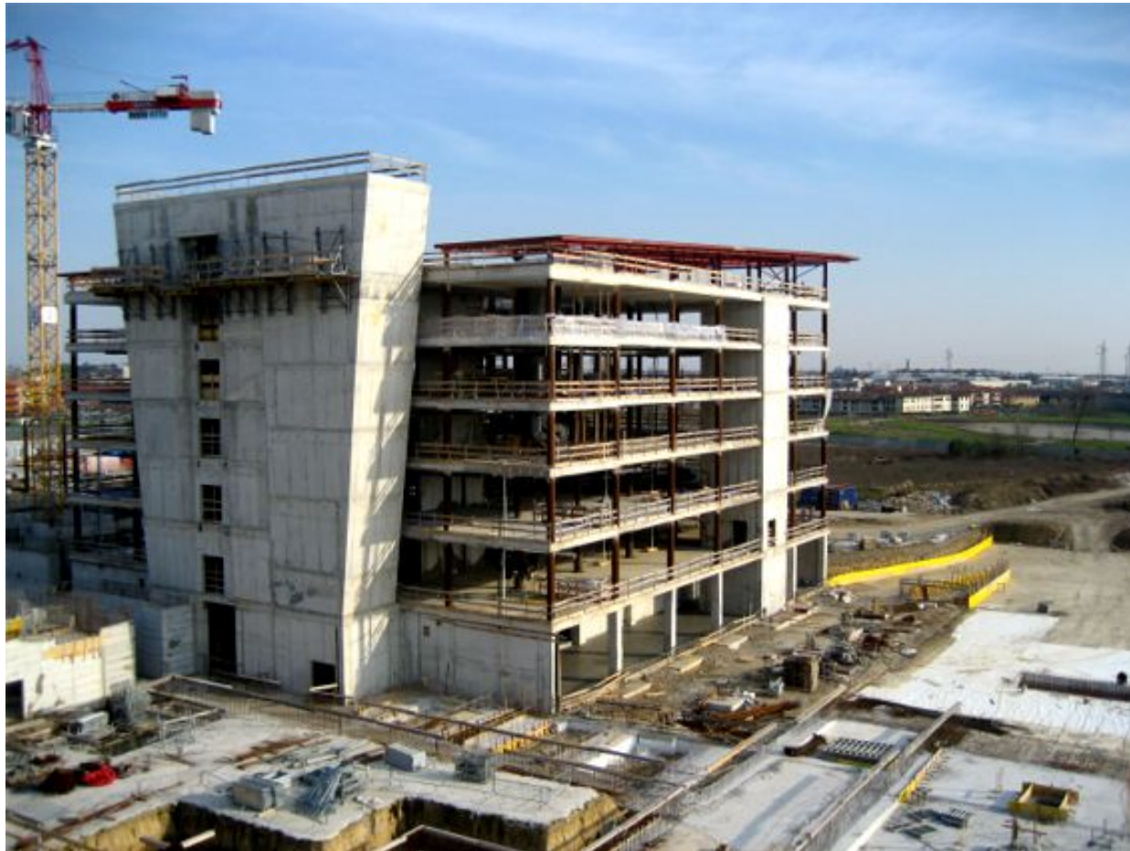
22/03/2007 Torre 1 e Hospital Street
